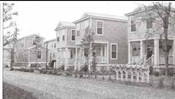
The Cottages at Oak Park in Ocean Springs was awarded a Platinum Level Leadership in Environmental Design Certificate on Thursday.
